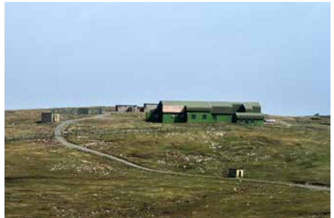
The surviving ROTOR period buildings at RAF Aird Uig.
